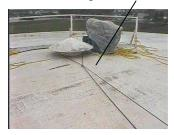
Caution- The center stand pipe must be structurally sound and capable of handling 1000 lb. pull at the base. The standpipe must be located in the center of the tank. If it isn't special cable connections must be made. Call RBW for help in set-up.
