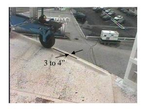
Place the fixture on the roof of the tank with the front tires about 3 to 4" from the edge of the tank. Make sure that the fixture is sitting square and that the rear of the fixture is pointed toward the center of the tank.
