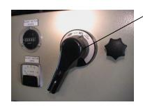
**Disconnect Switch**Turns power on and off
