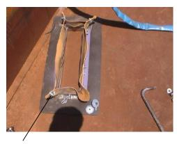
Clamp corners of the frame seal with 3/8" bolts And large washers as shown.
